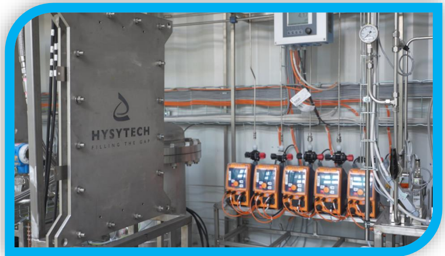
Figure 3 Electrochemical reactor of 0.2m 2 of electrode area for the CO 2 conversion
